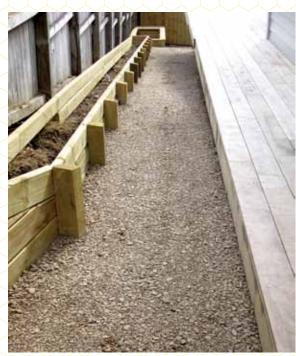
Step 5: A topping layer is recommended above the top of the JakMatEnviro, compaction is done with a plate compactor ensuring a sound and professional finish
